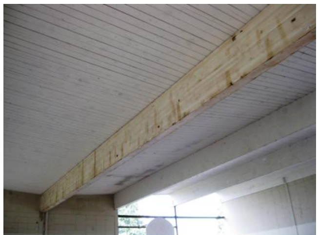
PI-ST-08 BEAM DRY ROT REPAIR
