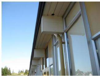
LH-ST-11 BEAM DRY ROT REPAIR Repair of dry rot at exterior wood beams needed to protect against further damage and deterioration.
