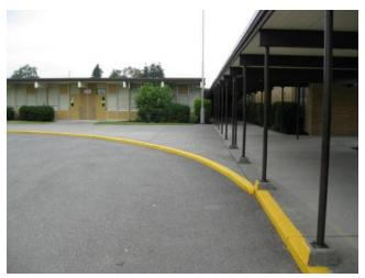
LH-SI-10 CURB RAMP ADDITION A curb ramp is needed at the front entry for wheelchair access and to meet ADA requirements.
