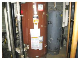
LH-ST-07 MECHANICAL EQUIPMENT ANCHORING Mechanical equipment needs to be anchored in place for seismic support.
