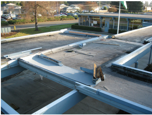
Temporary roofing installed at walkway roof to protect new roof decking.
