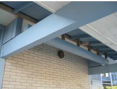
Temporary beam installed to support roof while work above is completed.
