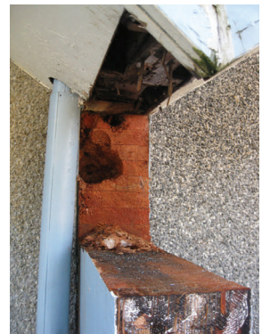
Deteriorated wood removed from the beam ends.
