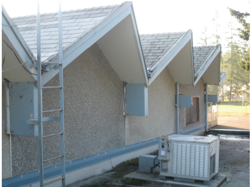
Downspouts removed from beam ends and deteriorated portion of beam ends removed.
