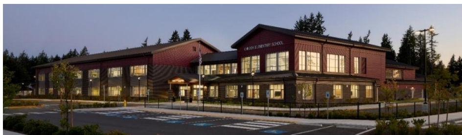
Chinook Elementary School - Built 2021
