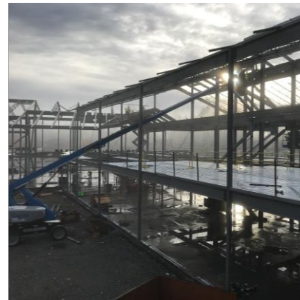
Chinook Elementary Steel Erection - 2022
